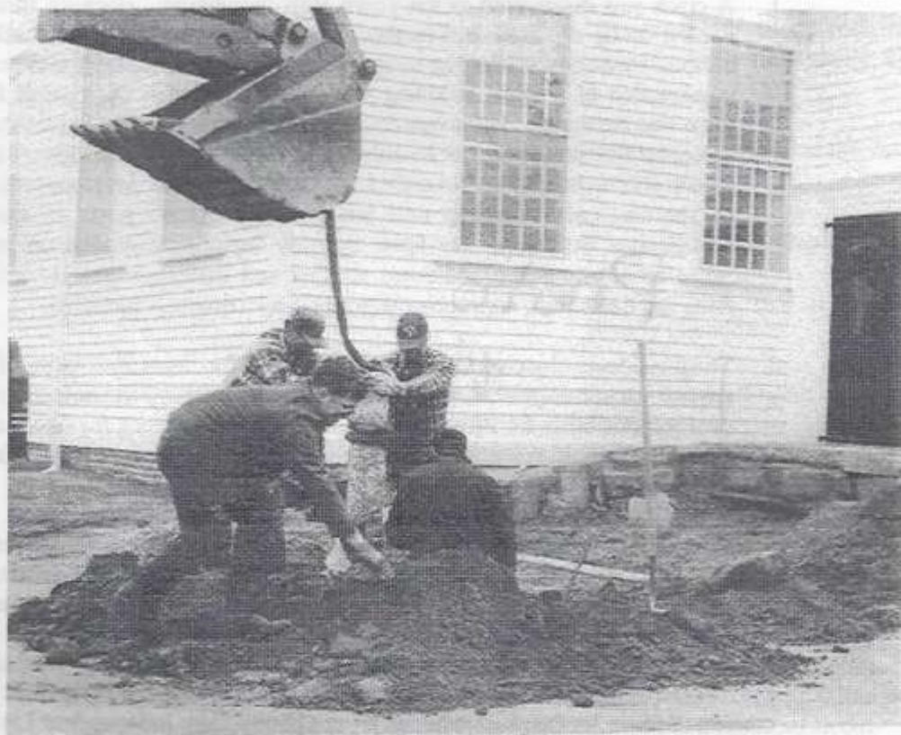
Highway Department installing ADA handicapped ramp at the Town Hall.
